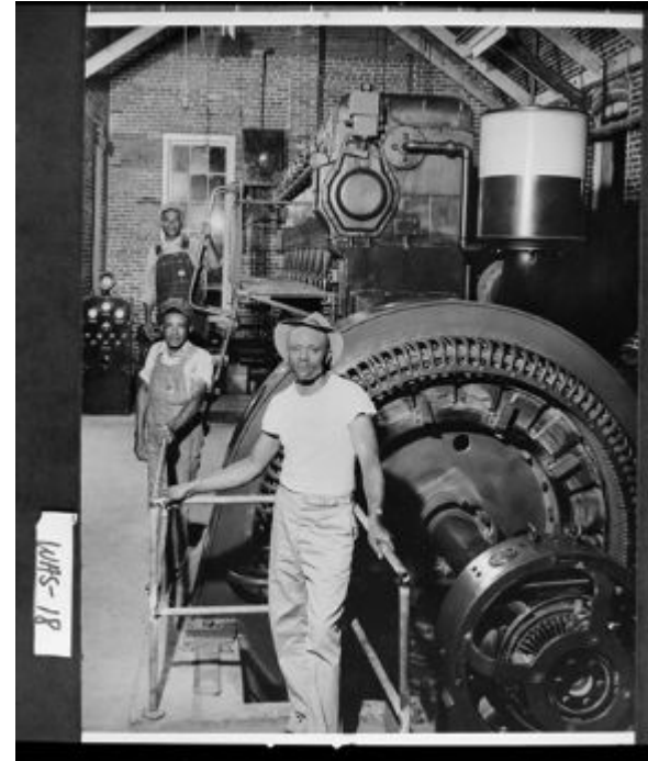
Sandersville, early 1940s. Workers seen standing beside the diesel engine and generator used by the city to produce its own electricity, Vanishing Georgia, Georgia Archives
