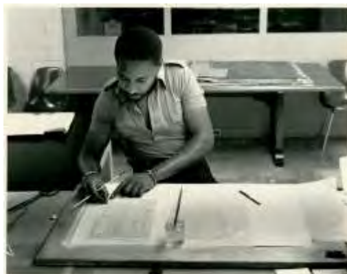
L-R: Deacidifying a document by sponging on magnesium carbonate (ca. 1975), sandwiching documents between layers of cellulose acetate and lamination film (1979), laminating sandwiched documents (1979). 4-1-57.
